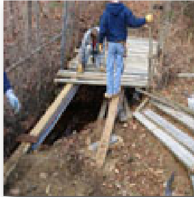
The New Bridge at Greenwater Pond
